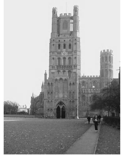
Fig. 12.2 A real case of broken symmetry: the mirror symmetry of the west front to Ely cathedral was lost when the north tower collapsed.
